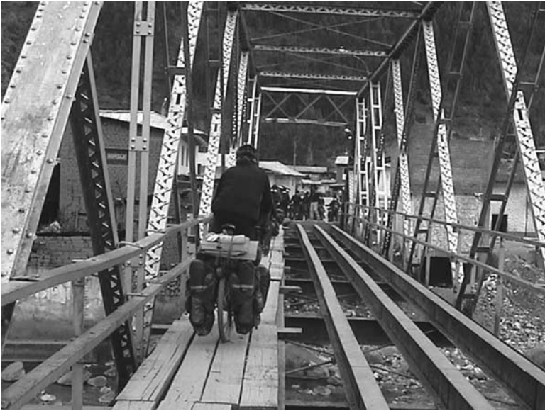
Tim crossing a dilapidated bridge.
