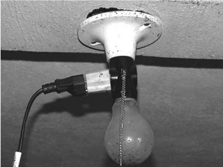
We used a T Adaptor to convert a light socket into an electrical outlet.
